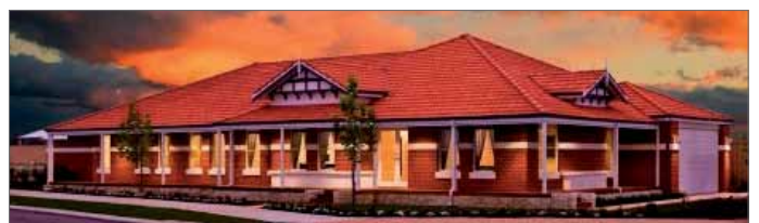
FIGURE 4: Example of a dwelling that addresses both the primary and secondary street through the use of gables, verandas, awning windows, and feature render and window sills (Source: Plunkett Homes, 2009)
