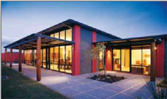
FIGURE 5: Example of skillion-roofed house with two visible separate and distinct planes. (Source: WA Country Builders, 2009)
